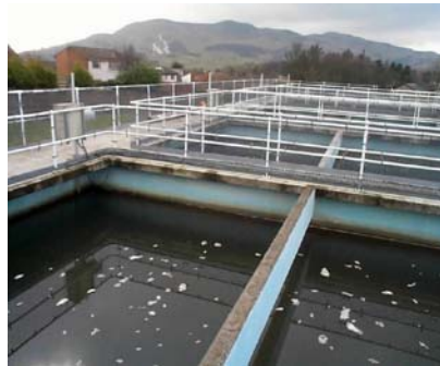
Rapid Gravity Filter (RGF)
